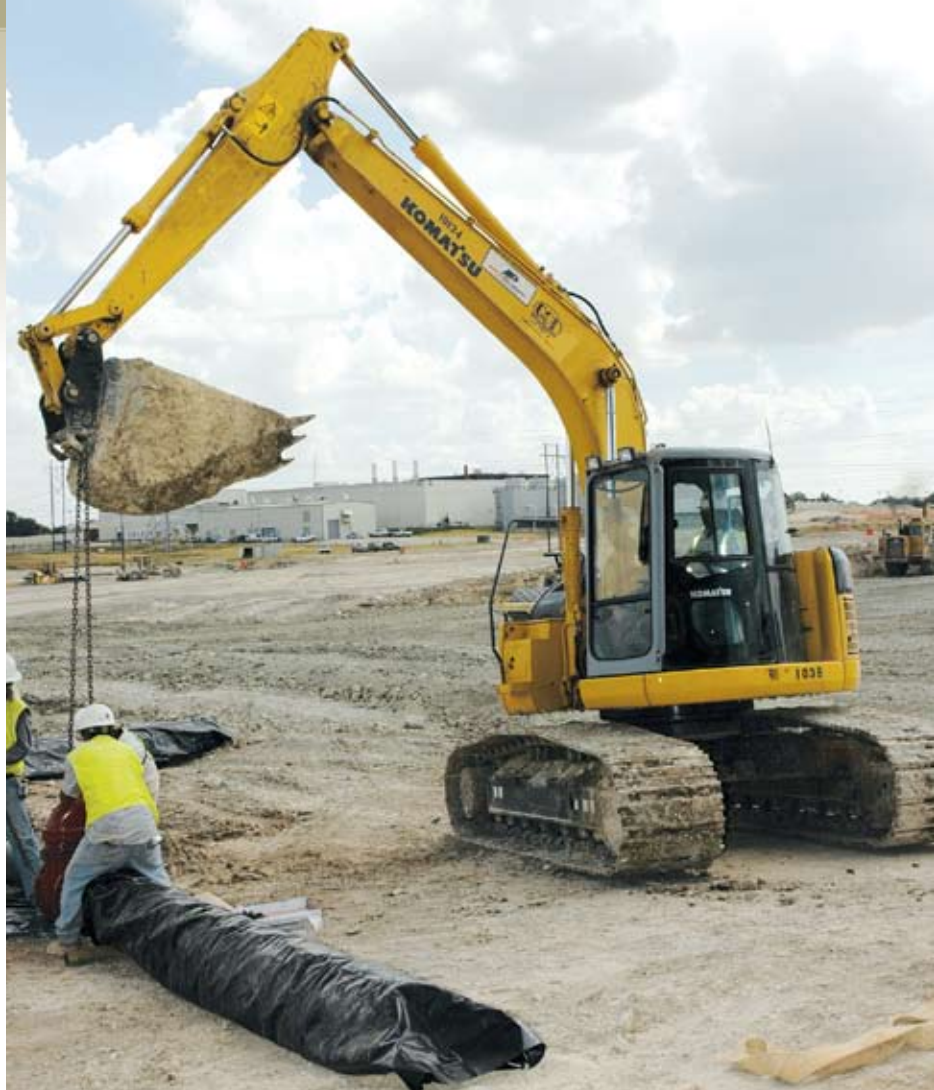
A Commercial Consolidated crew uses a Komatsu PC158USLC-2 excavator to dig trenches and set water pipe on a commercial development property in Austin.
