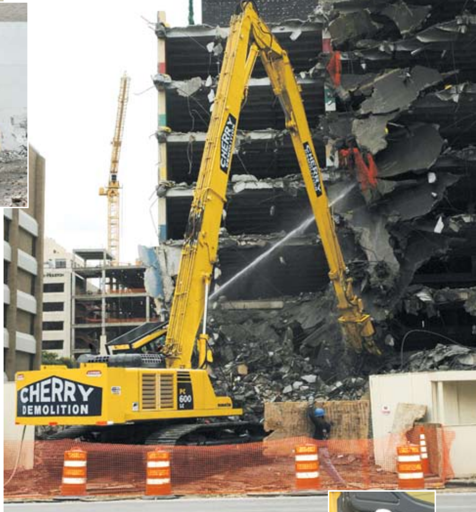
Samuel Huerta uses Cherry Demolition's new PC600LC-8 with LaBounty cracking jaws to take down part of the parking structure at the former Methodist Hospital in the Houston Medical Center. Cherry Demolition customized the machine with a camera and video monitor, a tilting cab, extra counterweight and an on-board water system for dust control. "I can tell the productivity on the high-reach application is better," said Huerta of the new machine, which features Komatsu's ecot3 Tier 3 engine. "I'm able to take more material down in less time, and that will benefit us in the long run."
