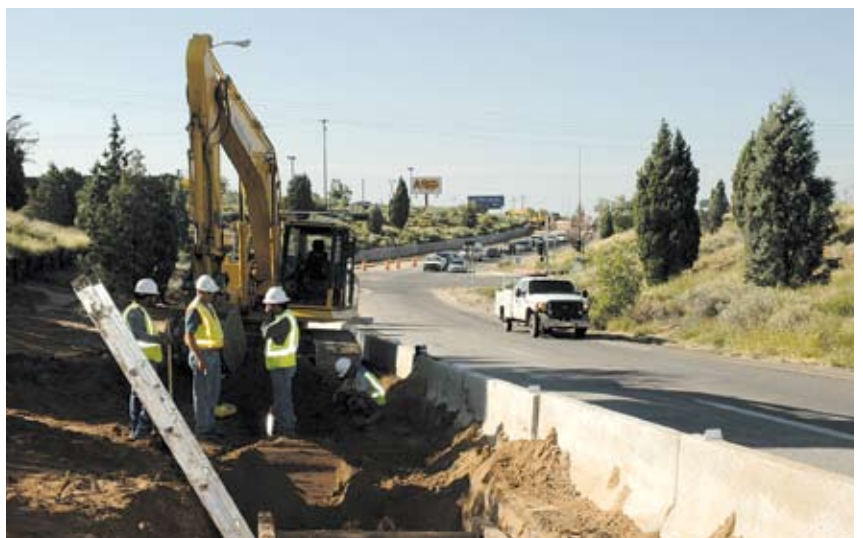
Underground contractors know good practices in trench safety are extremely important, including trench shields or boxes for deep excavations, ladders for egress at proper intervals and hard hats and other safety gear to keep workers protected from potential falling objects.
