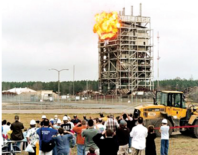
An initial blast starts the implosion process on an industrial plant demolition that D.H. Griffin performed in 2006.
