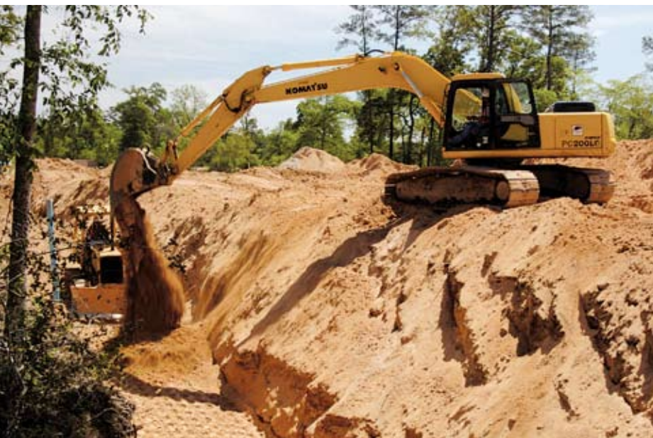
A Triple B Services operator backfills a ditch using a Komatsu PC200 excavator, one of the staples in the company's fleet.
