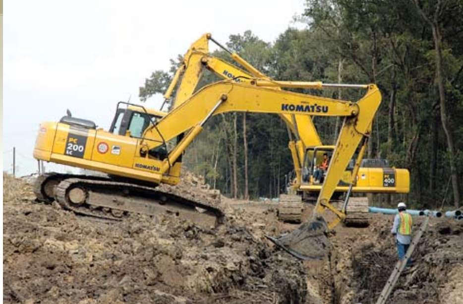
Komatsu excavators play a large role in Triple B Services projects. "The excavators offer us versatility because we can use them for clearing, digging trenches and setting pipe in utility work and digging and loading during mass excavation," said Co-owner Keith Burke.
