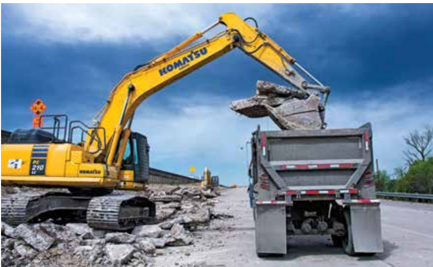
Operators perform pavement removal from roadways, parking lots and more with Cherry Companies' Komatsu excavators.
