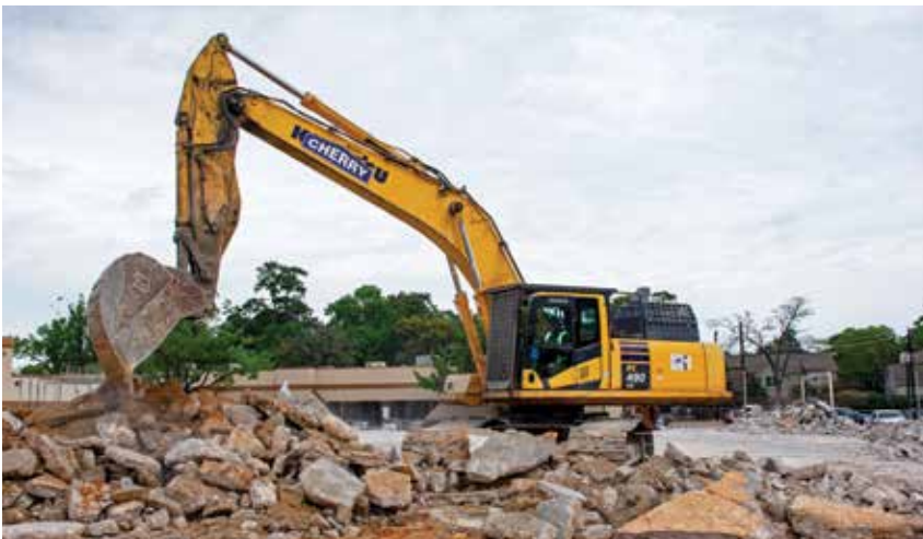
Operators perform pavement removal from roadways, parking lots and more with Cherry Companies' Komatsu excavators.
