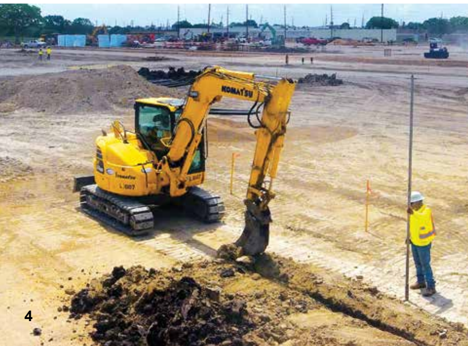
A Linco Construction Co. Inc. operator digs a utility trench with a Komatsu PC88MR excavator while a laborer checks grade.
