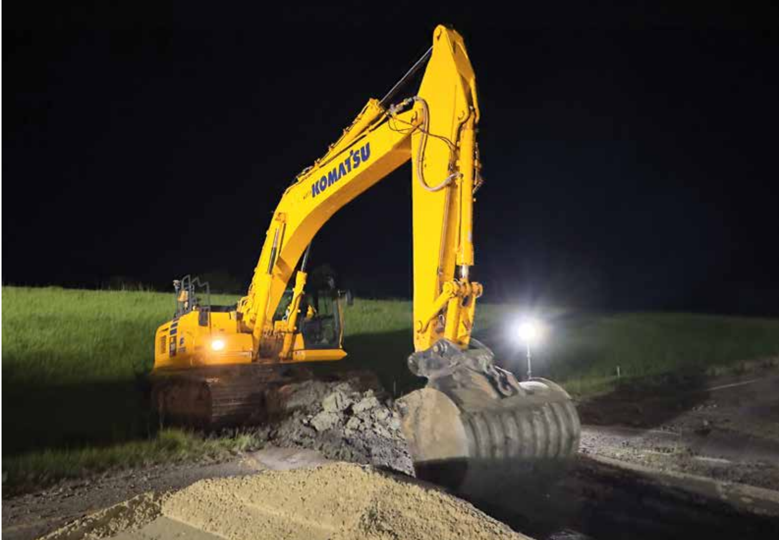
Operator Jose Revera digs a trench with a Komatsu PC360LCi-11 Intelligent Machine Control (IMC) excavator. "The GPS is helpful for getting to target grade and not going past," said Revera. "The excavator is strong and fast. It has good power, so I can lift pipe and boxes with no issues."
