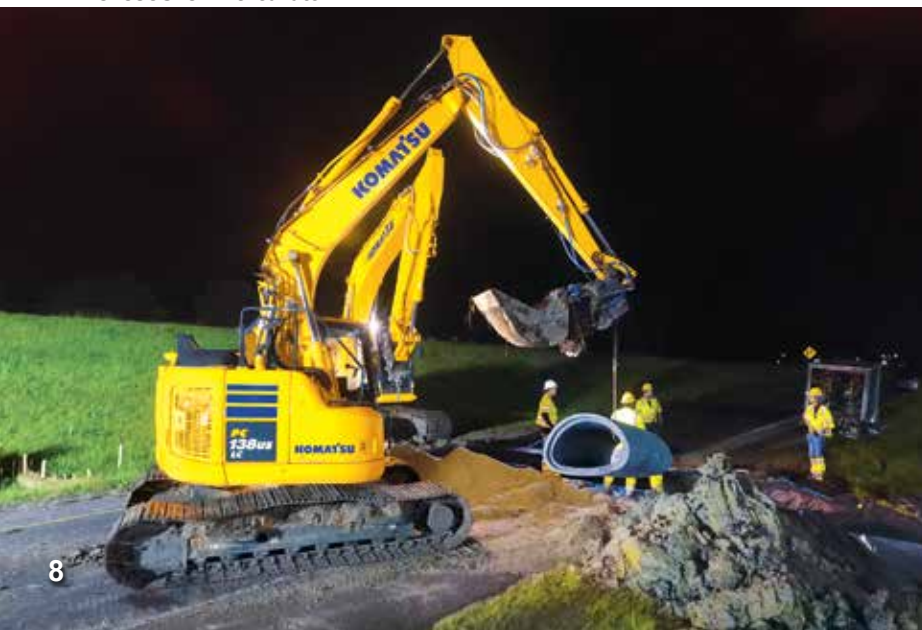
Gascot Construction lowers concrete storm pipe into a trench with a Komatsu PC138USLC-11 excavator.
