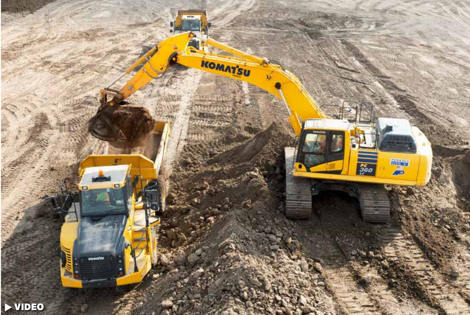
Perkins Civil operators move material with a Komatsu PC360LC-11 excavator and rented Komatsu haul trucks.
